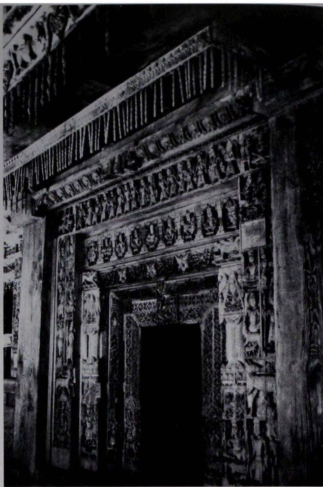
Fig. 30 Multiple door frame of Hiḍimba Devī temple, Manali
