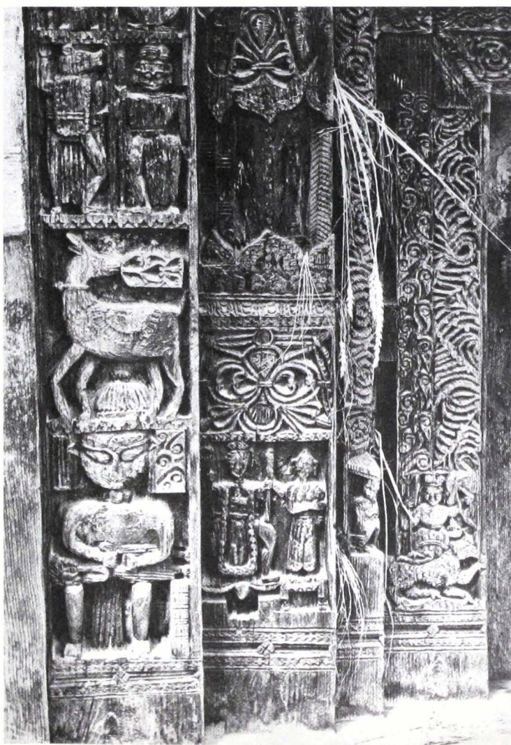
Fig. 19 Detail of multiple door frame, Gautam Rishi temple, Goshal, Kulu
