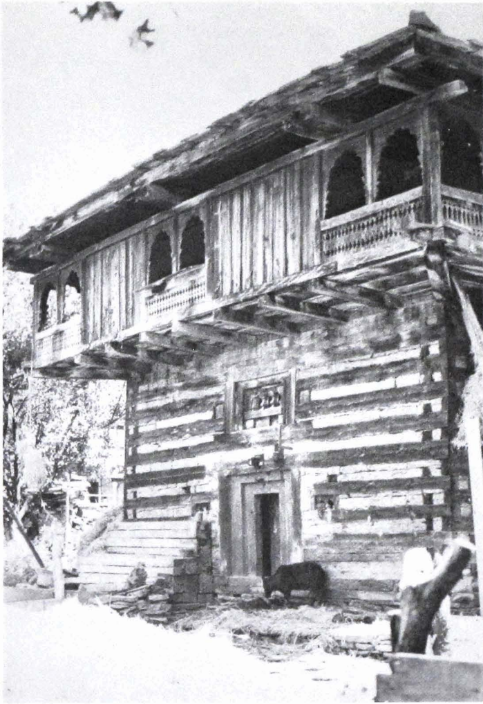
Fig. 23 House in Dashed village, Kulu valley
